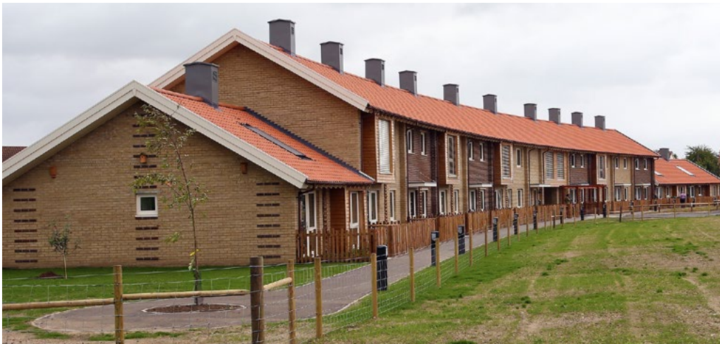
Fig 69: Ditchingham Passivhaus, Hastoe (Credit: Hastoe Housing Association)
