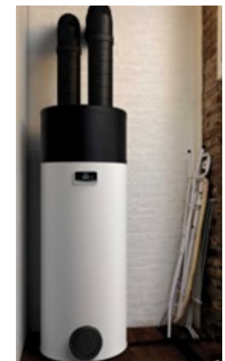
Fig 67: Example DHW HP installation (credit: Vaillant)
