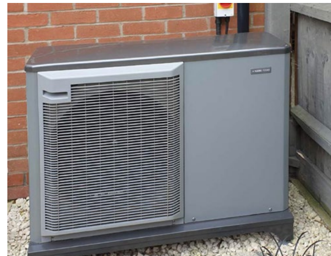
Fig 66: Example ASHP outside unit (credit: Dr J Wingfield)
