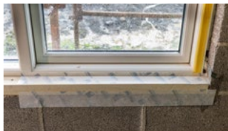
Fig 83: Taped junctions (credit: Ecological Building Systems)
