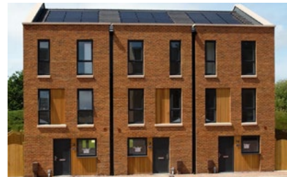
Fig 22: Example of homes built to similar standard as CS2a (credit: VerdeGO Group)
