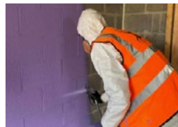
Fig 84: Liquid VCL being sprayed (credit: Intelligent Membranes)
