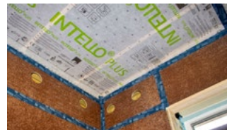
Fig 85: Taped airtight board (credit: Ecological Building Systems)
